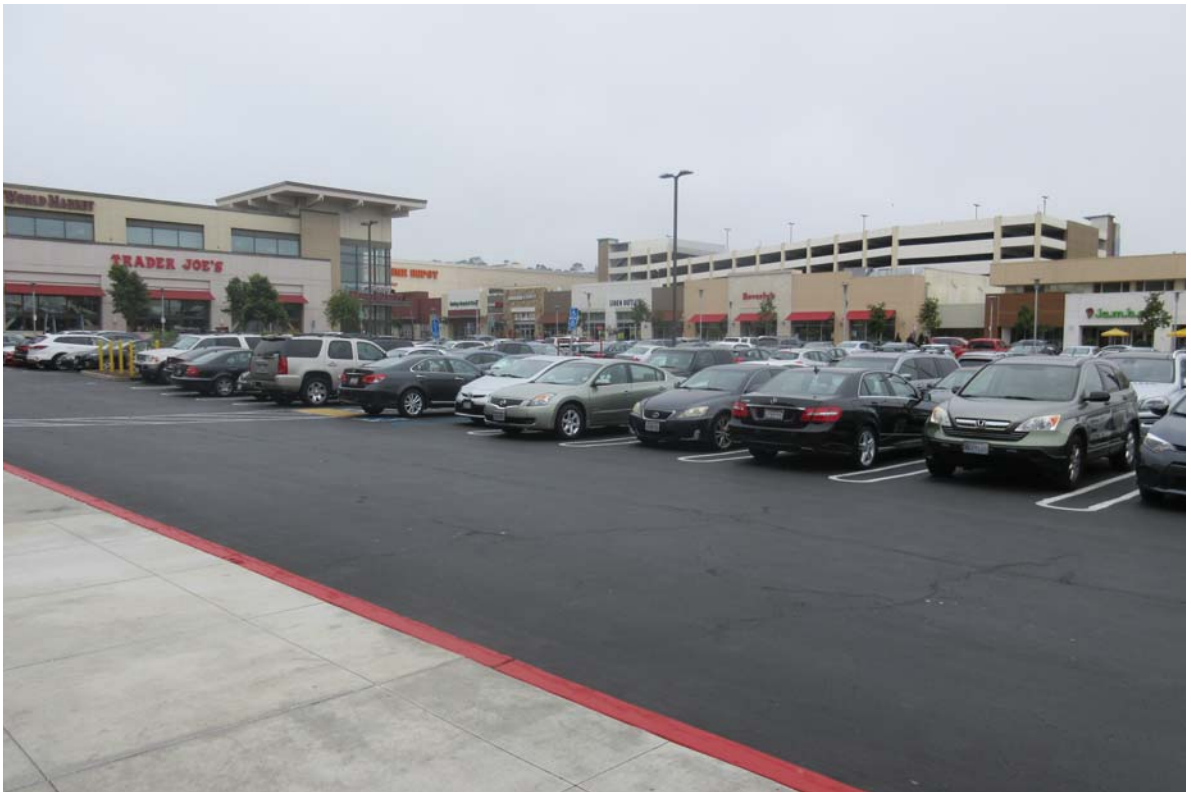
PHOTO 3: View of retail development west of project site looking from existing surface parking in the Westlake Shopping Center.
