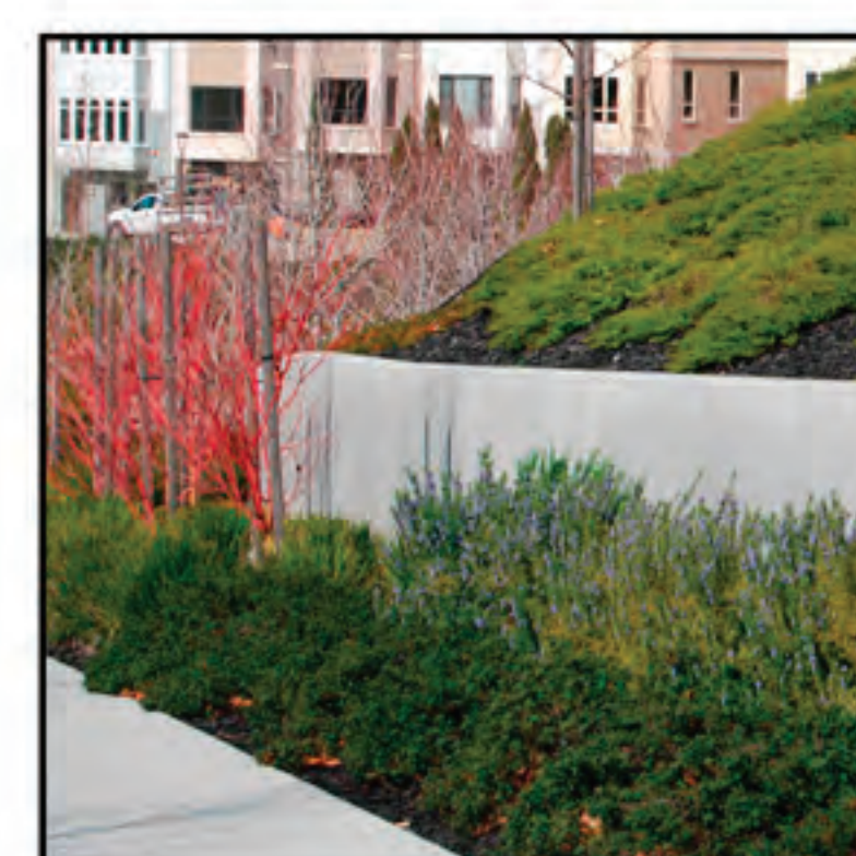
Concrete Retaining Wall
