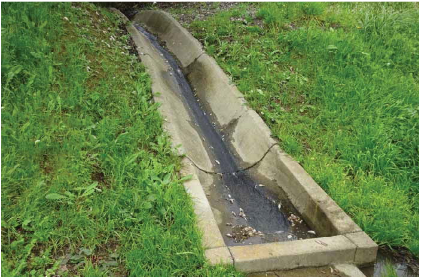
12. View of drainage swale discharging runoff to storm drains on Steve Courter Way, east property.
