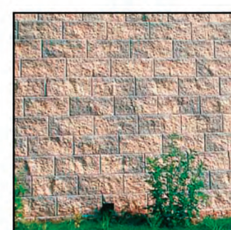
Block Retaining Wall
