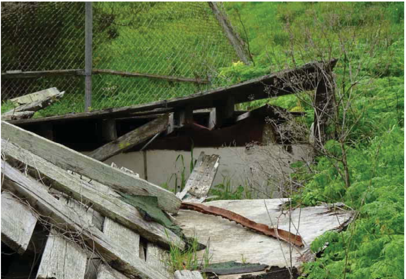
7. View of demolition debris pile with visible empty 55-gallon drum, east property.
