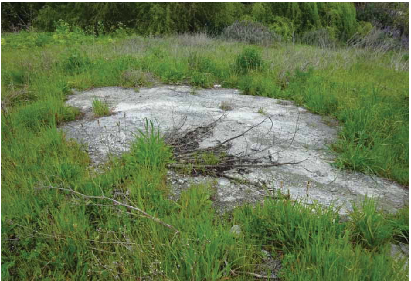
2. View of abandoned concrete pad, northeast property.
