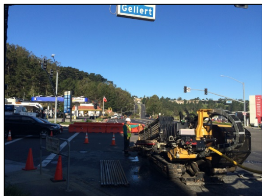
Serramonte Boulevard: Sewer main was replaced by reaming method, a trenchless technology that reduced traffic impacts.
