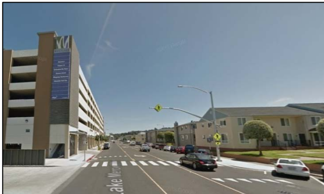
Lake Merced Boulevard: City leveraged private developer funds to construct bulb out, rapid flashing lights, and high visibility crosswalks.
