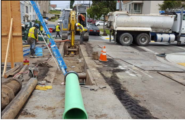
1 st Avenue: Sewer main was replaced in 2016.
