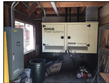
Fire Station 95: The outdated emergency generator was replaced with a safer, more efficient model capable of operating 8 times longer than the previous model.
