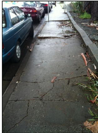
Schwerin Street: 2015-16 Annual Concrete Safety Project repaired sidewalk uplifted by street trees.
