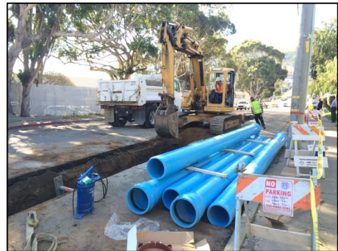
Schwerin Street: Water main replaced in 2015.
