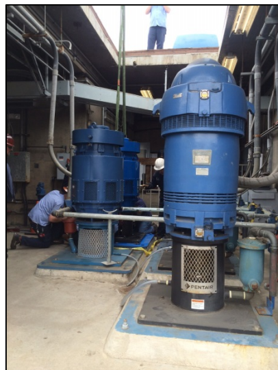
Wastewater Treatment Plant: Final effluent pump was replaced.
