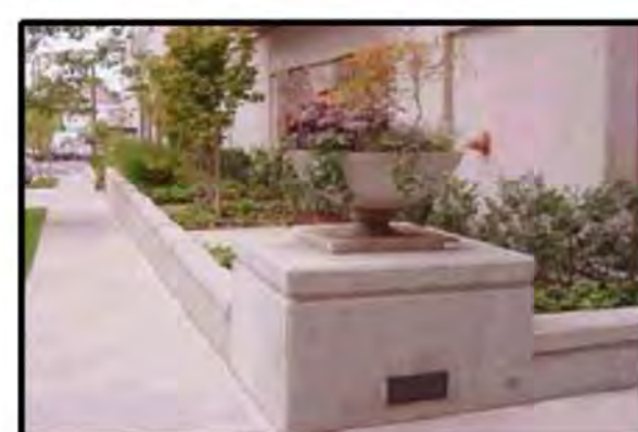
Precast Planters on Pedestal
