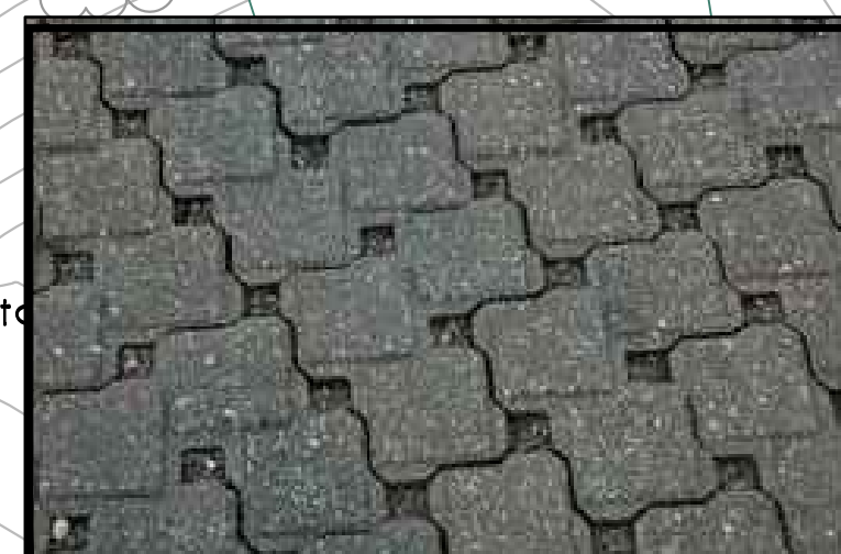
Permeable Entry Paving
