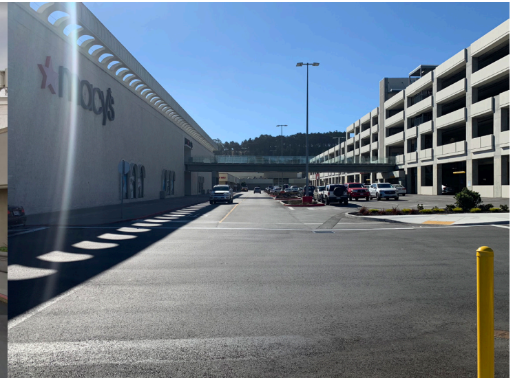
MALL ENTRY - LOOKING SOUTH
