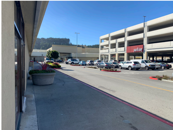
MALL ENTRY - LOOKING SOUTH
