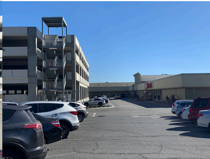
MALL ENTRY - LOOKING SOUTH
