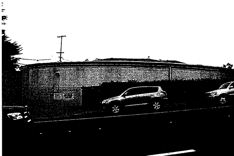
View looking east toward water tank
