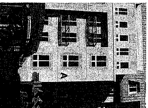
Exhibit 7B - Existing Building ID sign at Bldg. A
