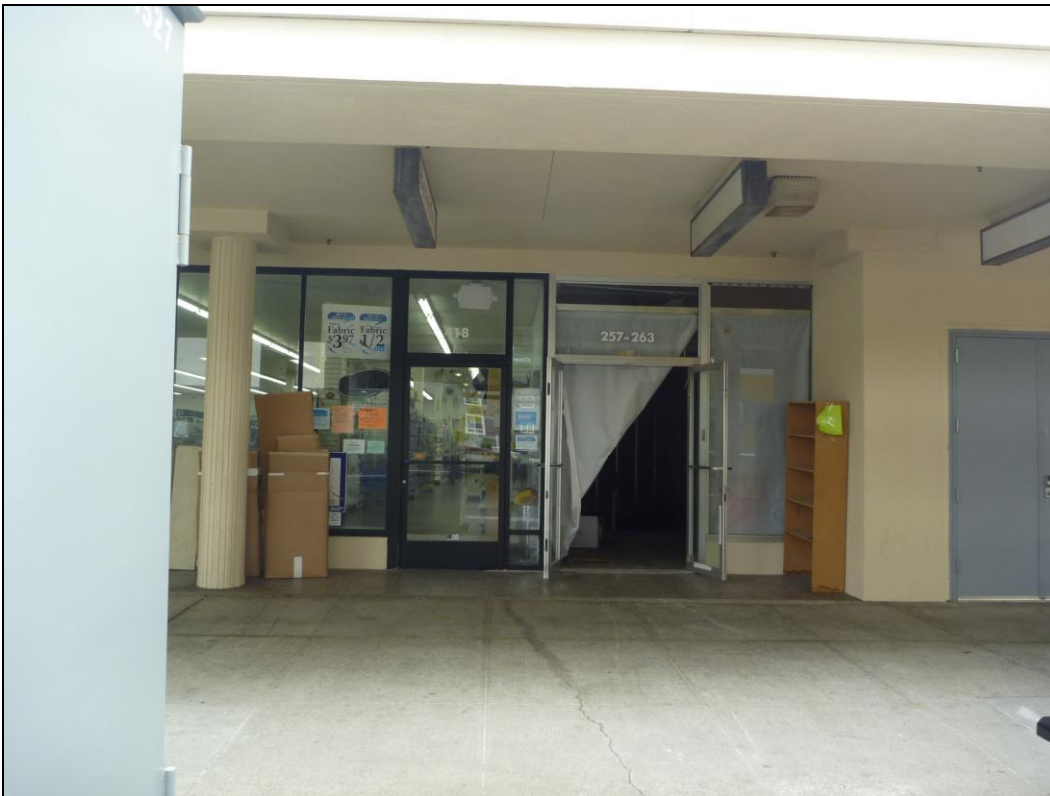
7 Description: Future entrance of Fitness 19/Rear of Beverly's.
