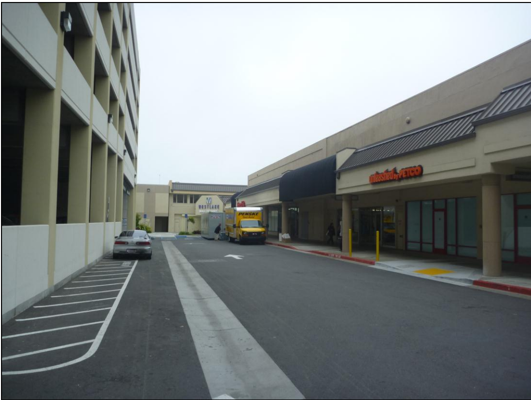
6 Description: Drive lane between Building S and parking garage. Facing north.
