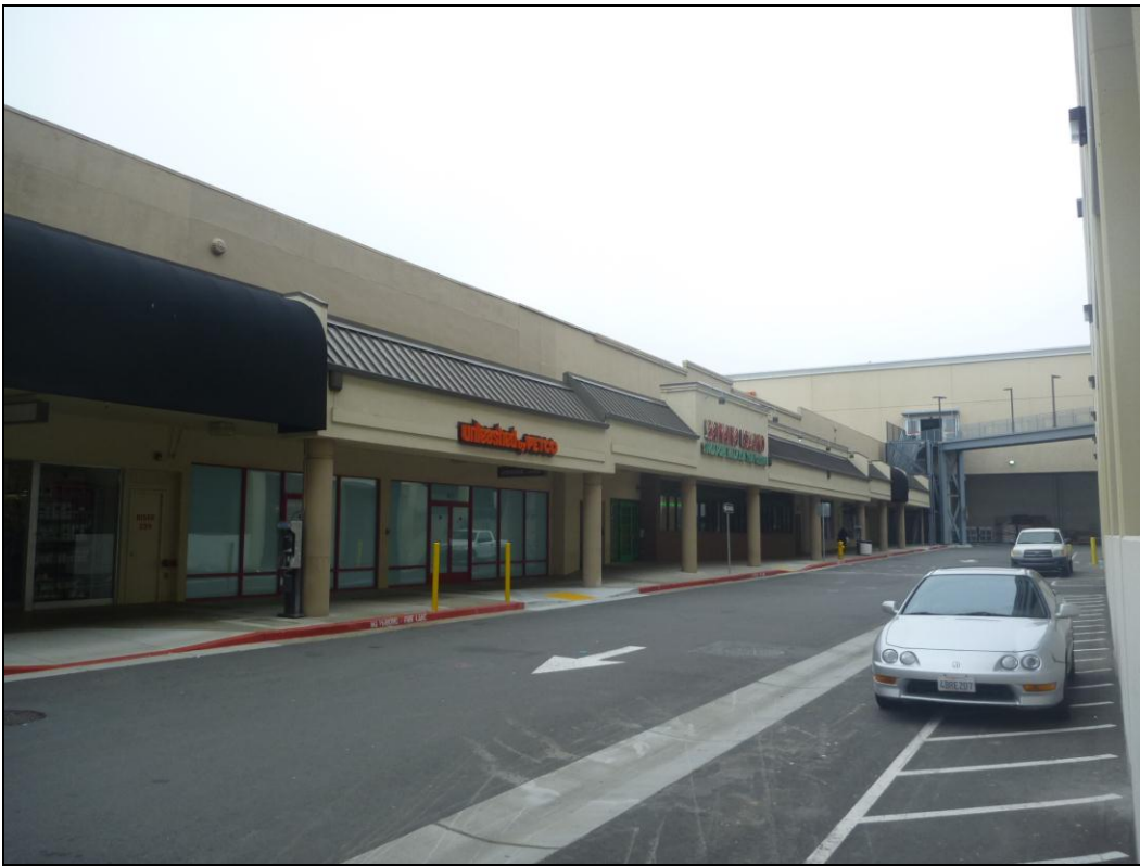
1 Description: Drive lane between parking garage and Building S. Facing south.
