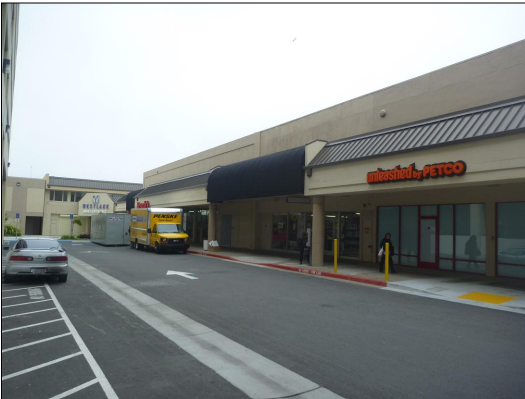
2 Description: Drive lane between parking garage and Building S. Facing north.
