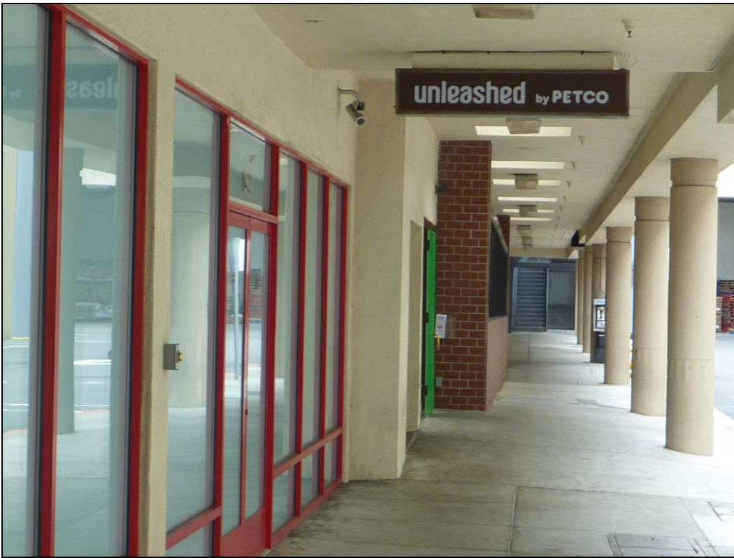
3 Description: Rear of Petco. Typical canopy signage.
