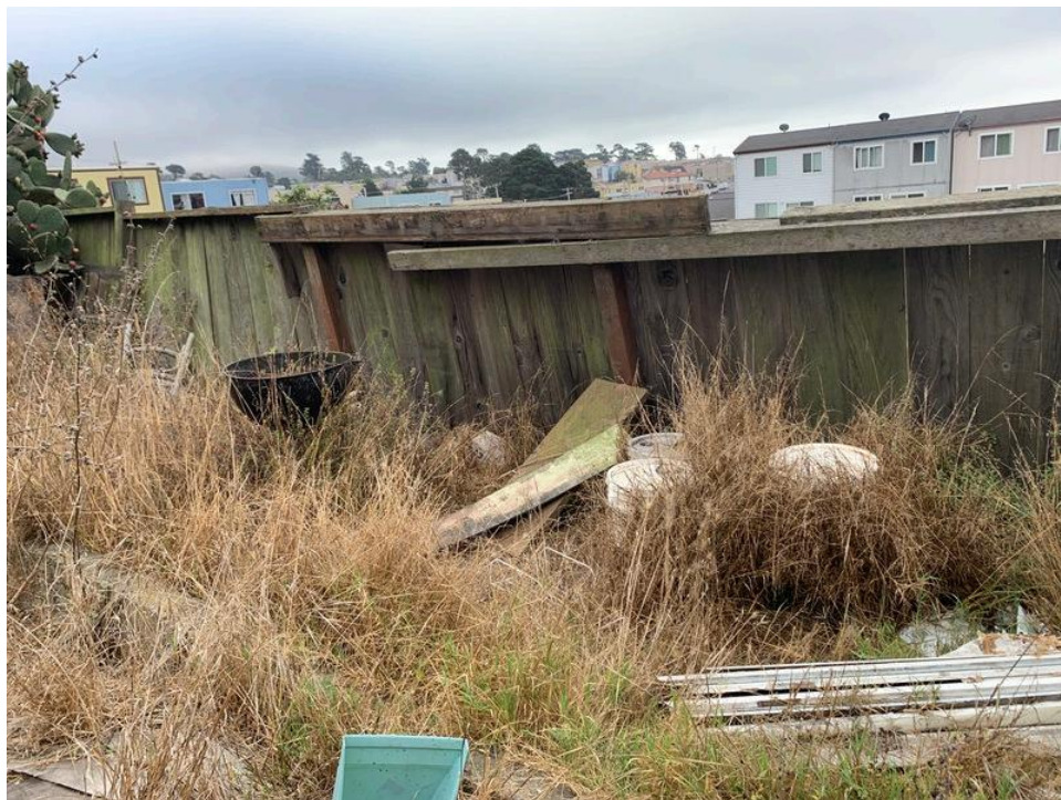
18. View of debris
