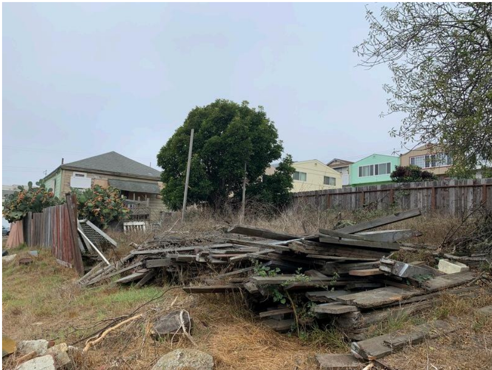
16. View of debris piles
