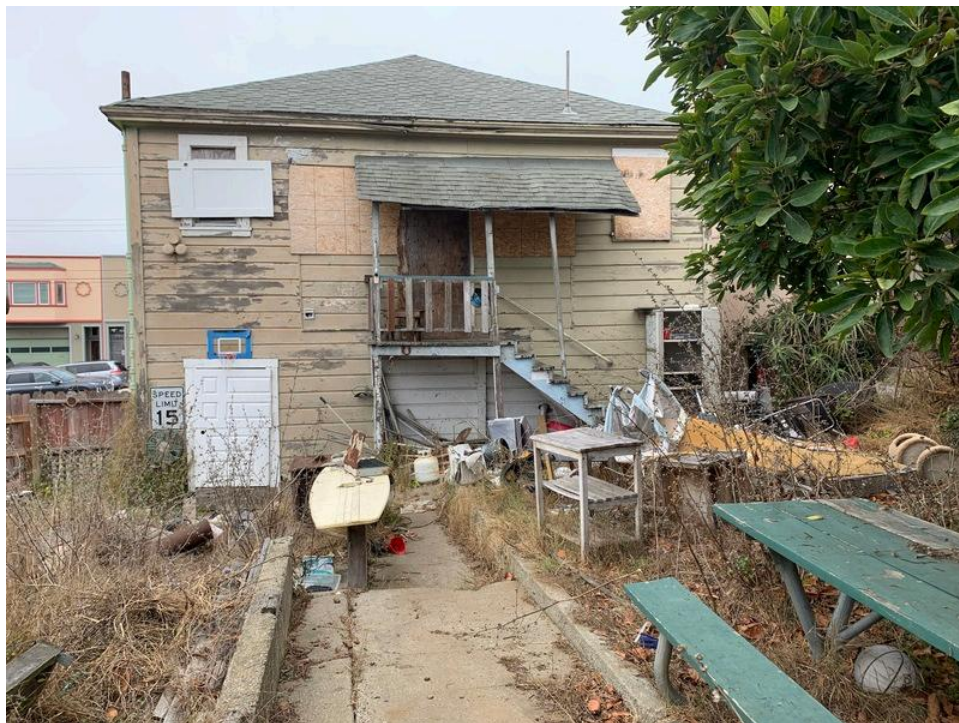
4. View of the west side of the residence, facing east
