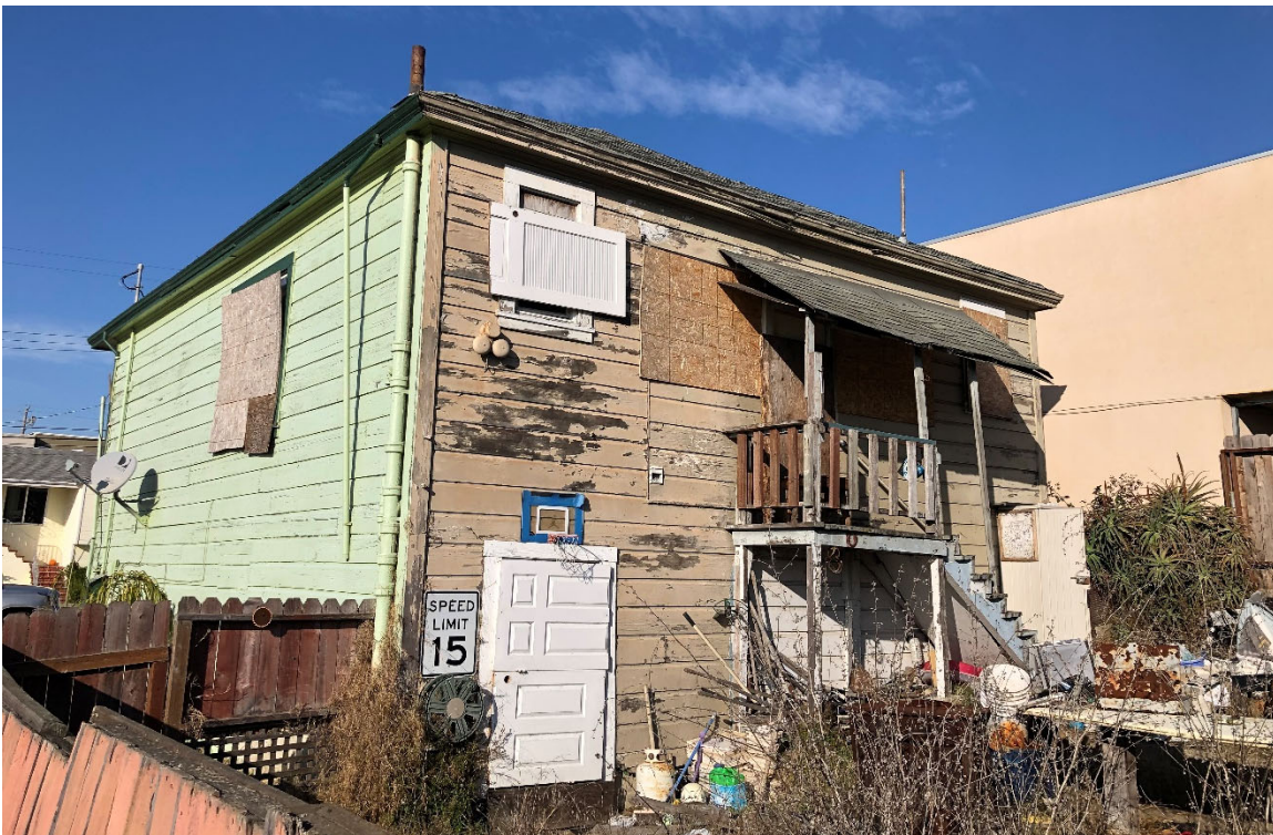
Figure 3. The rear (east) and south façades.
