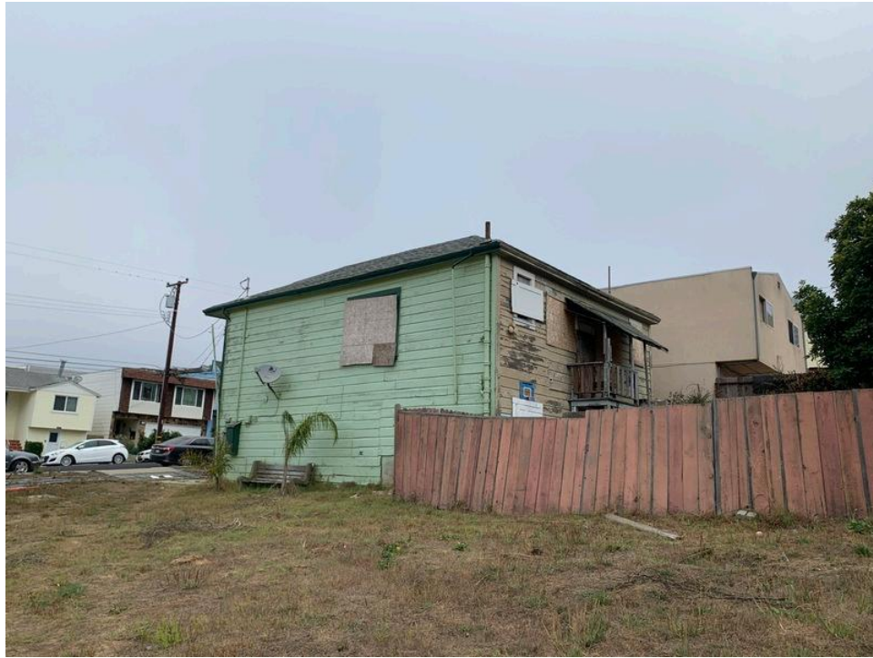
3. View of the south and west side of the residence, facing northwest
