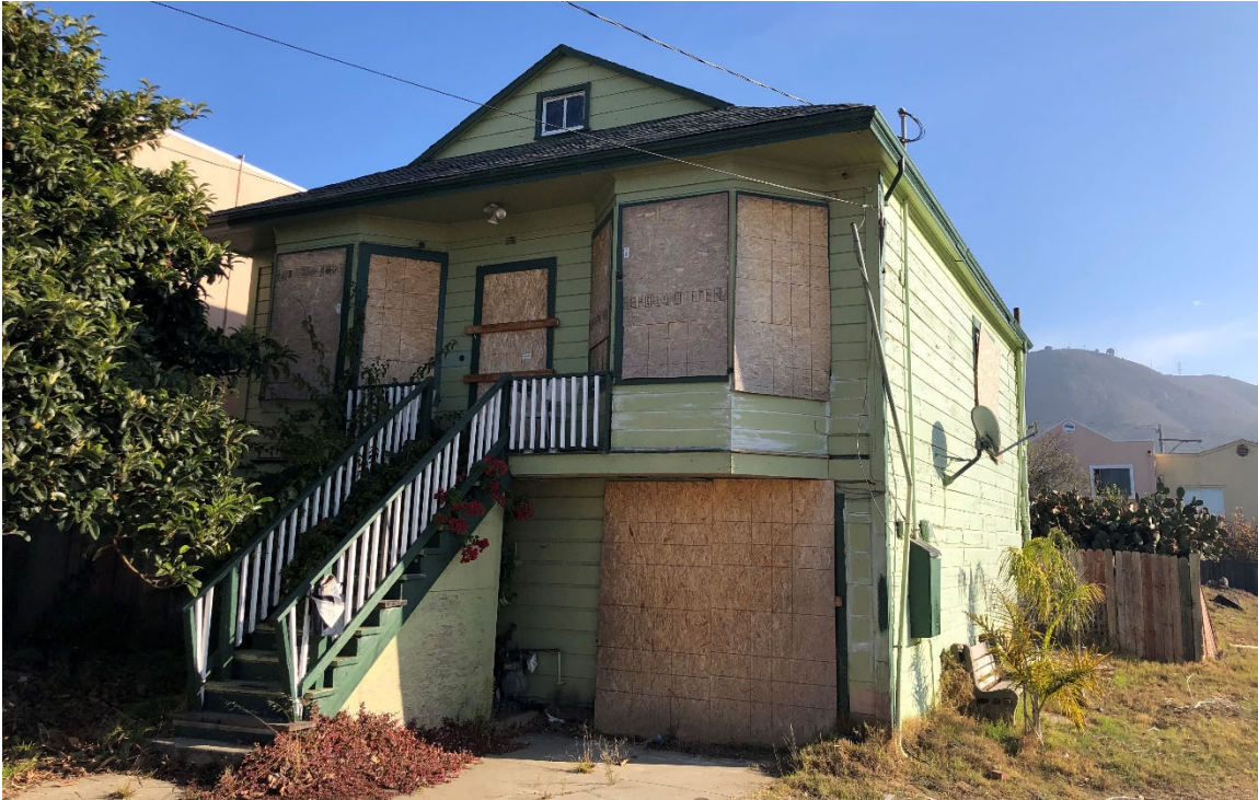
Figure 2. The front (west) and south façades of 141 3 rd Avenue.
