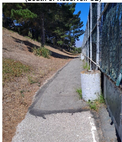
1-1d. Looking Northwest (West of Reservoir 5B)
