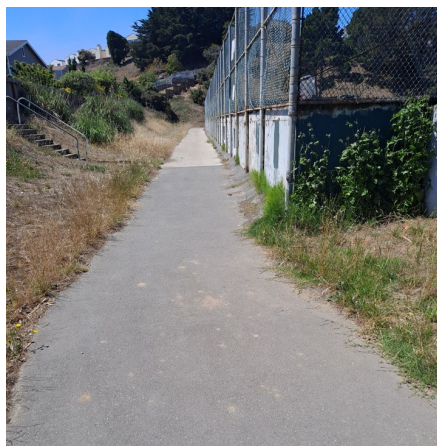
1-1a. Looking Southwest (South of Reservoir 5B)
