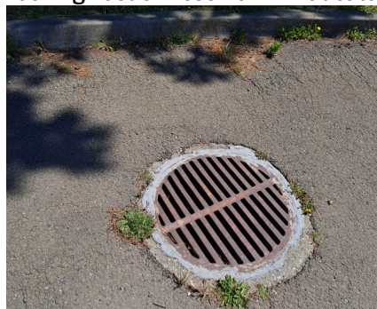
2-2f. Looking East of Reservoir 5 B at catch basin
