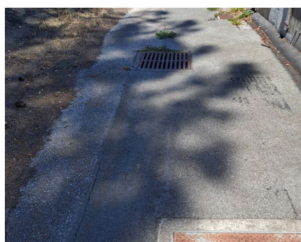
2-2b. Looking West of Reservoir 5 B at catch basin
