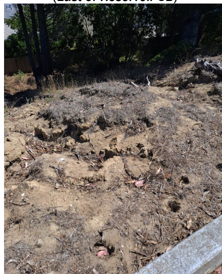
2-1d. Looking northeast downhill slope (East of Reservoir 5B)
