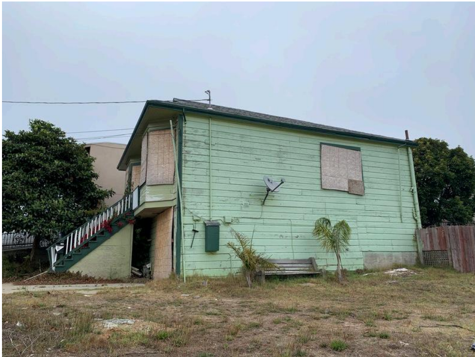
2. View of the south side of the residence, facing north
