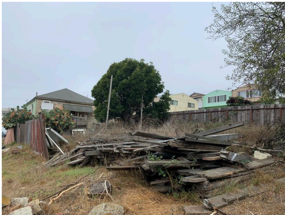
16. View of debris piles
