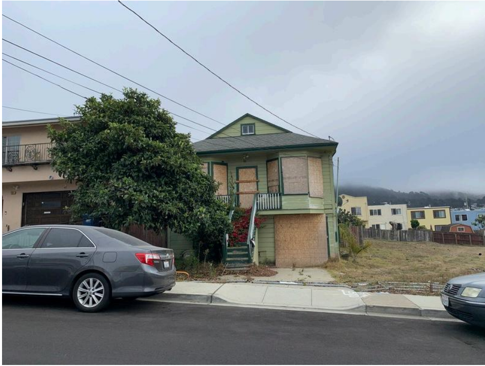
1. View of the subject property residence, facing east
