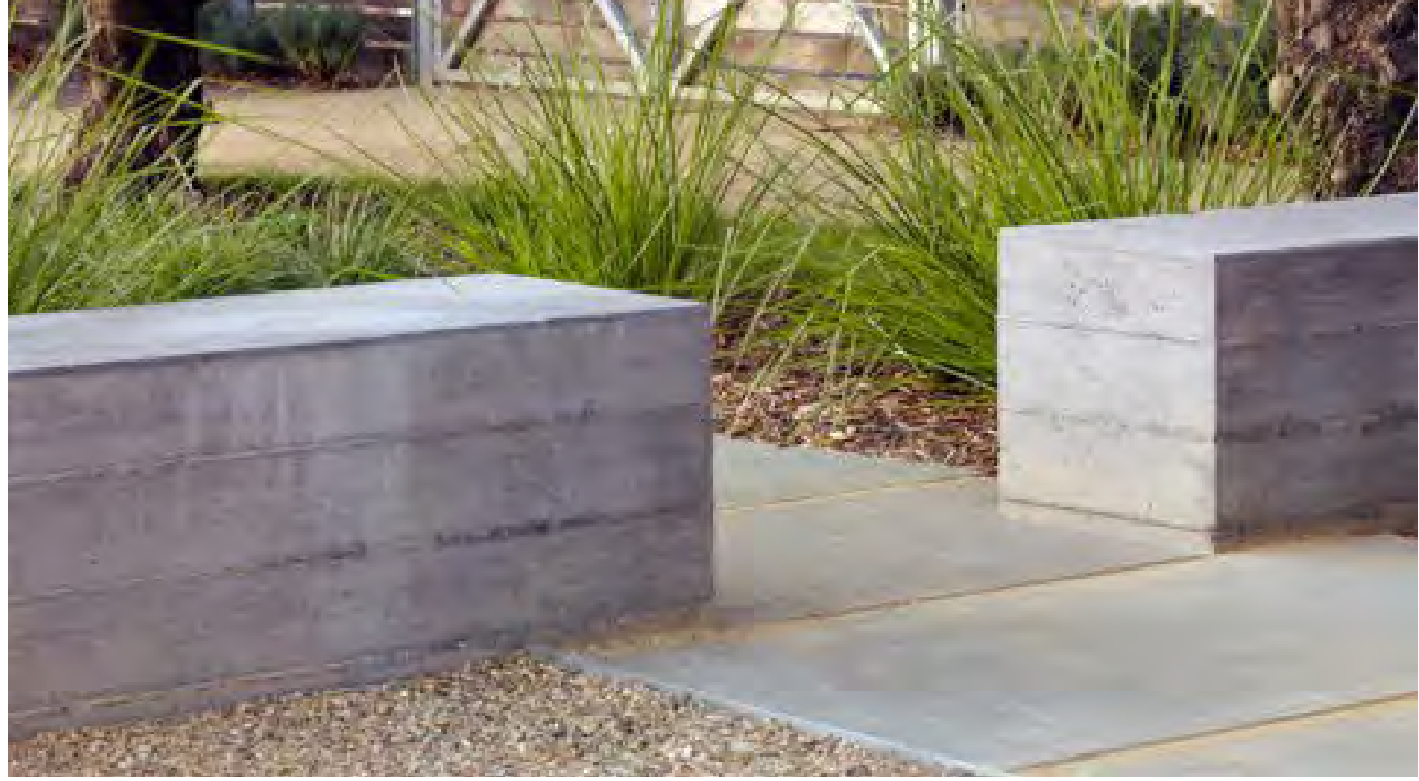
BOARD FORM CONCRETE WALL AT OVERLOOK PARK
