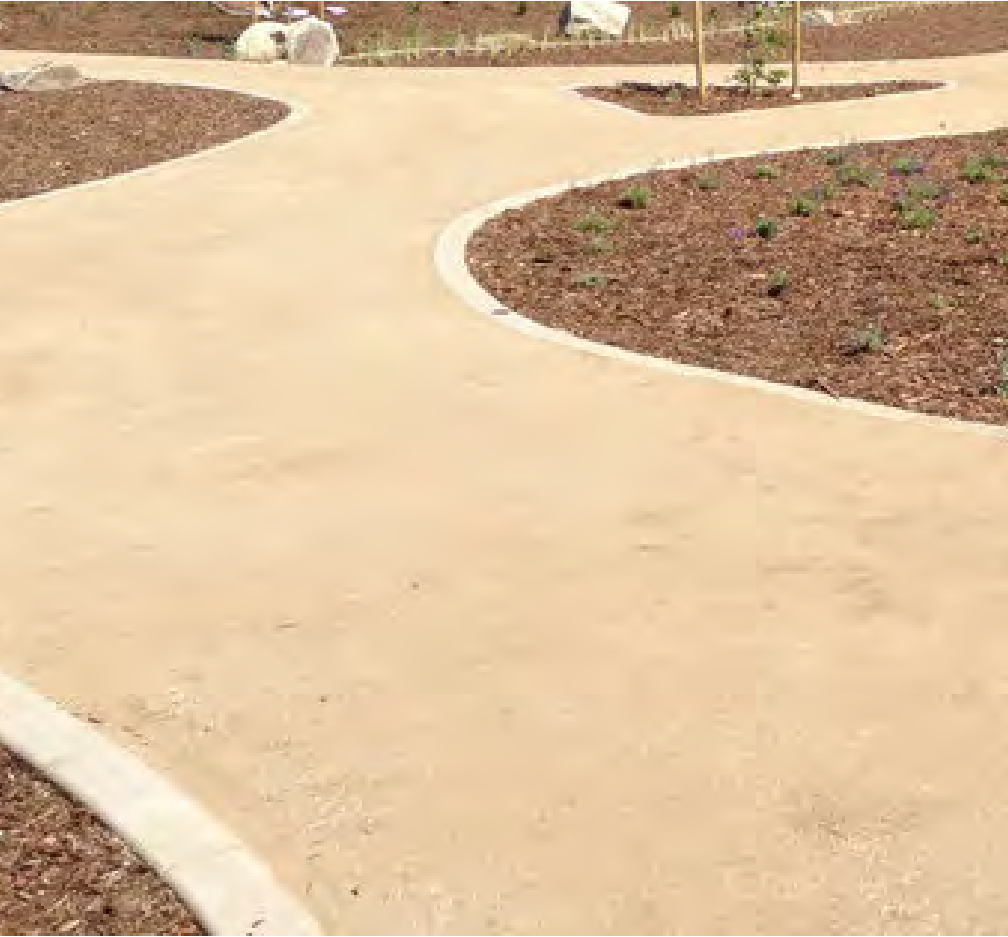
DECOMPOSED GRANITE PAVING AT COURTYARD RAISED PLANTERS
