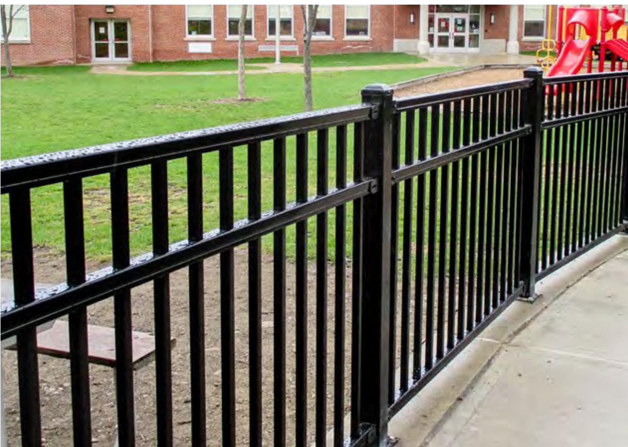
42" HIGH METAL ENCLOSURE FENCE AROUND PLAY AREA
