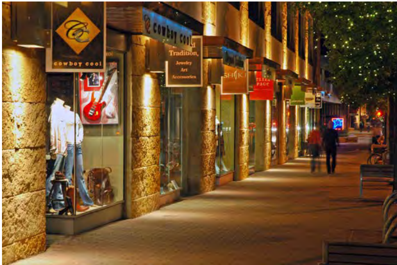
Luminaires highlighting a building facade.
