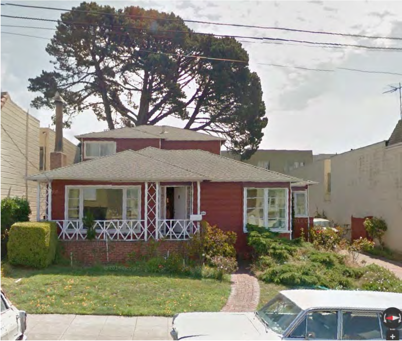
FRONT FACADE PHOTO SHOWING THE OLD TREE THAT FEEL ON GARAGE
